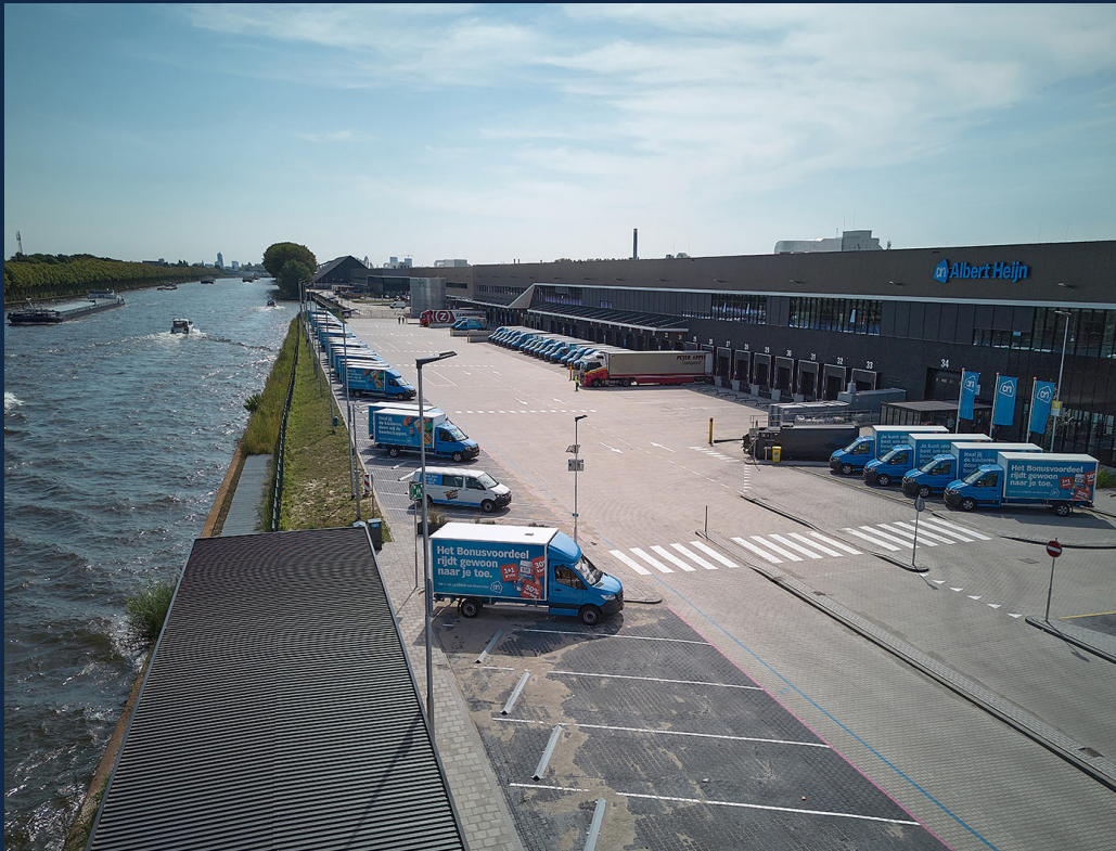
DISTRIBUTION CENTRE LAGE WEIDE | UTRECHT
