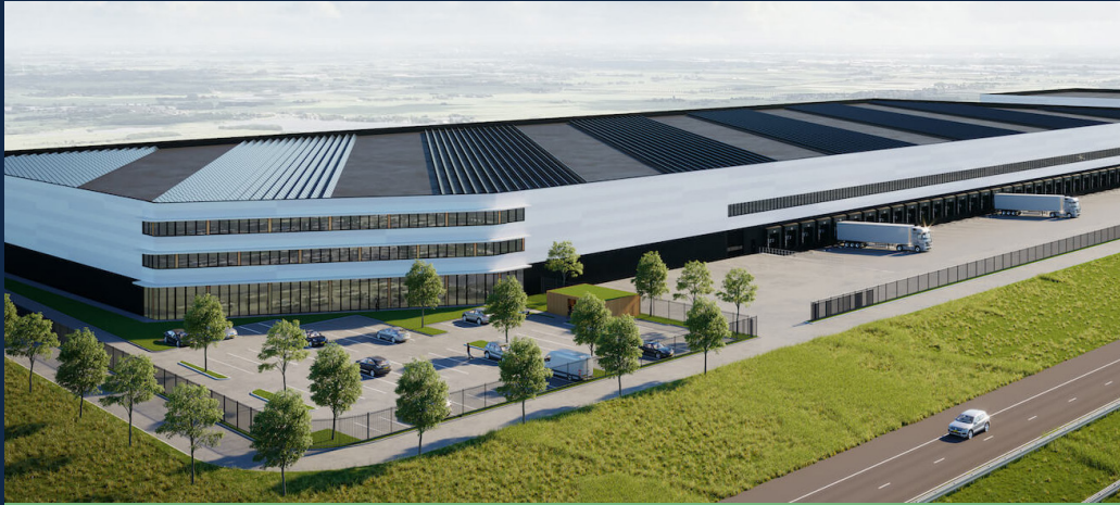
DISTRIBUTION CENTRE APELDOORN NOORD II | APELDOORN
