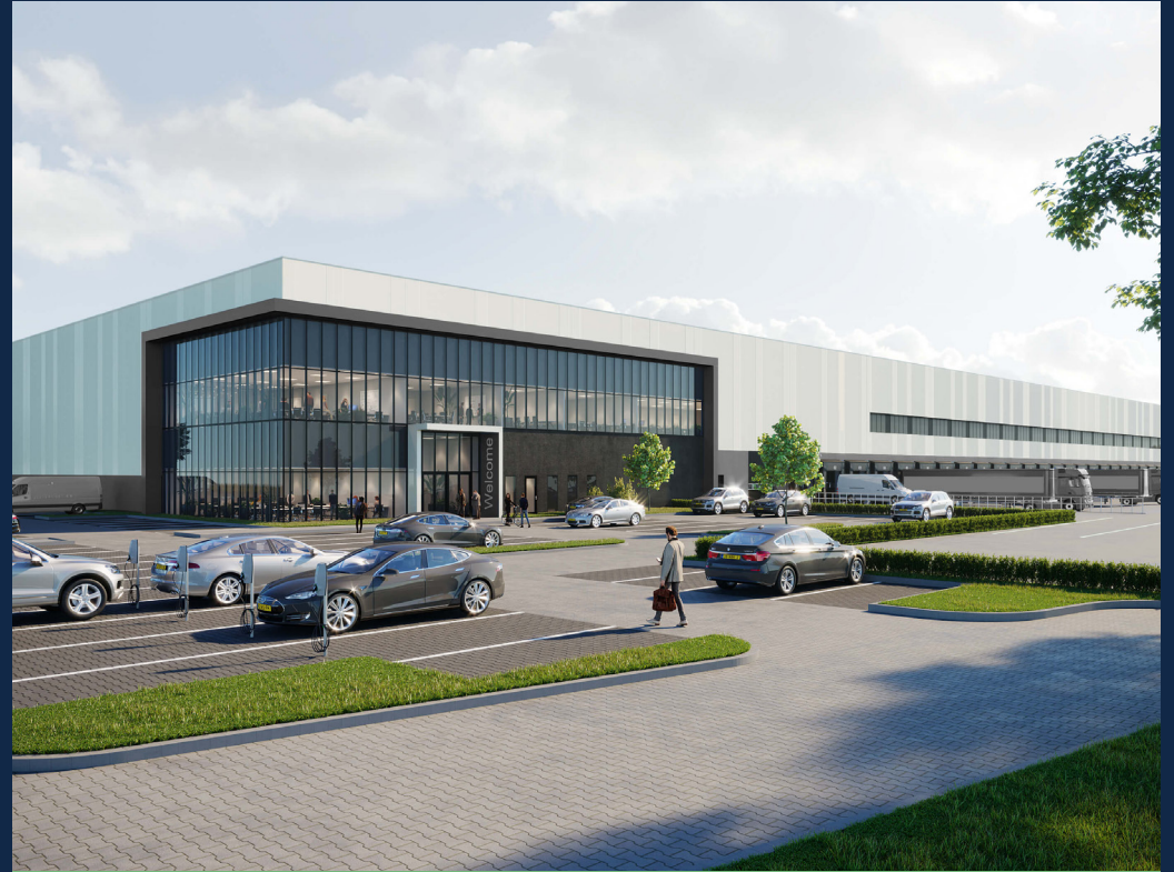
DISTRIBUTION CENTRE WILDEMAN II | ZALTBOMMEL
