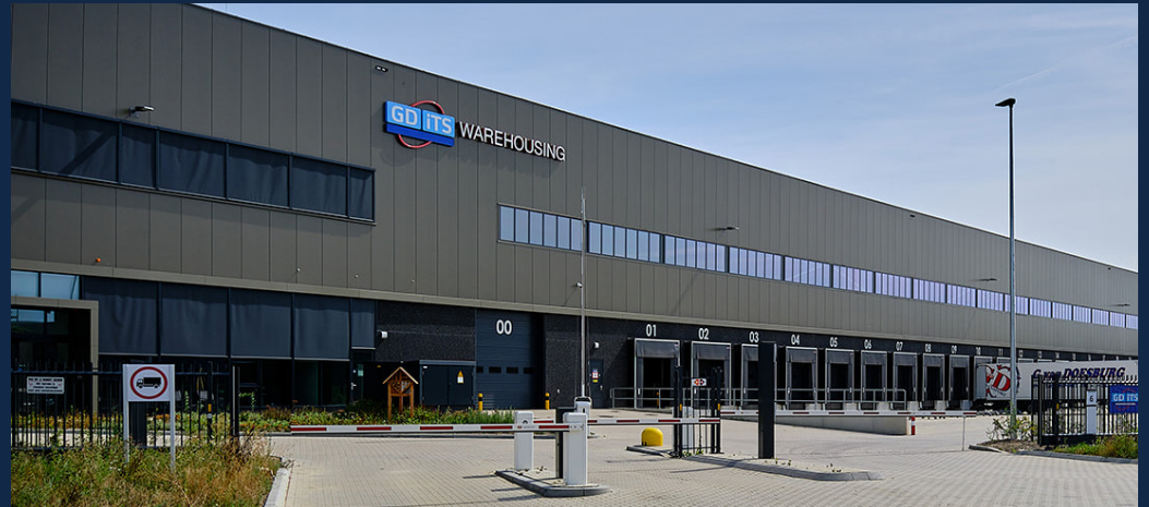
DISTRIBUTION CENTRE WILDEMAN II | ZALTBOMMEL
