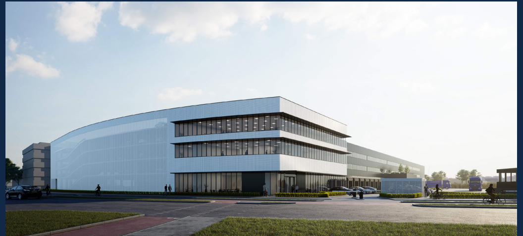
DISTRIBUTION CENTRE LAGE WEIDE | UTRECHT
