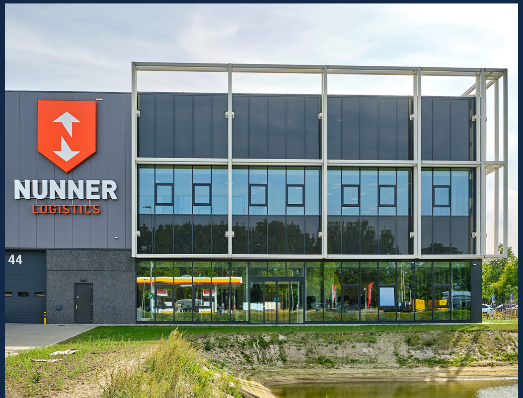
DISTRIBUTION CENTRE METAL VALLEY | DRUNEN
